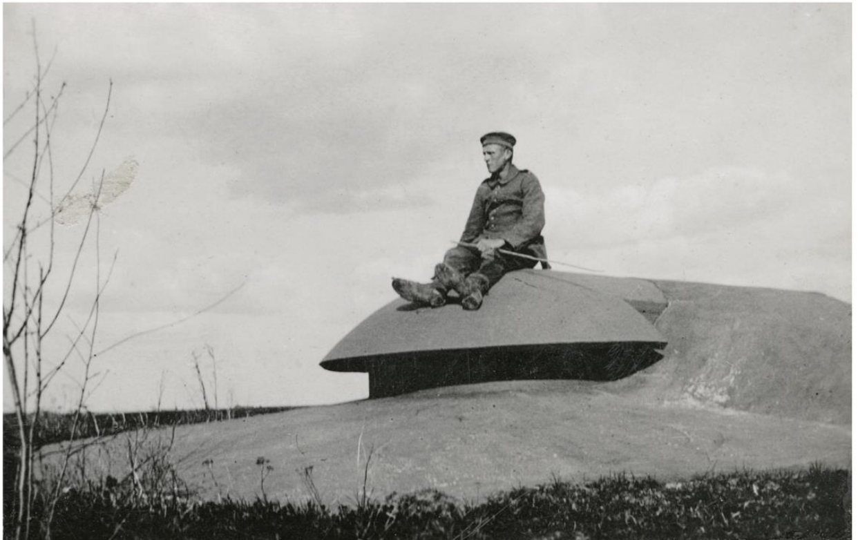
A German imperial soldier is sitting on the A. Ariens system armoured observation turret on the roof of the barracks of the Ninth Fort of Kaunas Fortress, 1915-1916. © Bayerisches Hauptstaatsarchiv
